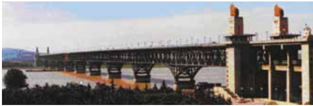
5. Nanjing Yangtze River Bridge, China.
