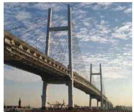
20. Yokohama Bay Bridge, Japan.
