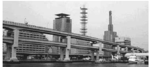
7. Shinko-Maya Elevated Road Bridge, Japan.
