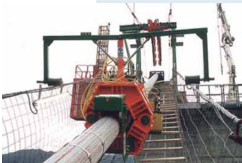
↑ Cable compacting
