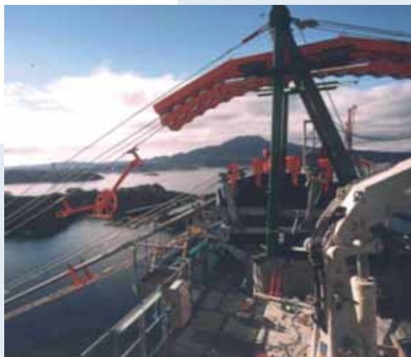
↑ Spinning wheel over de pyloontop
