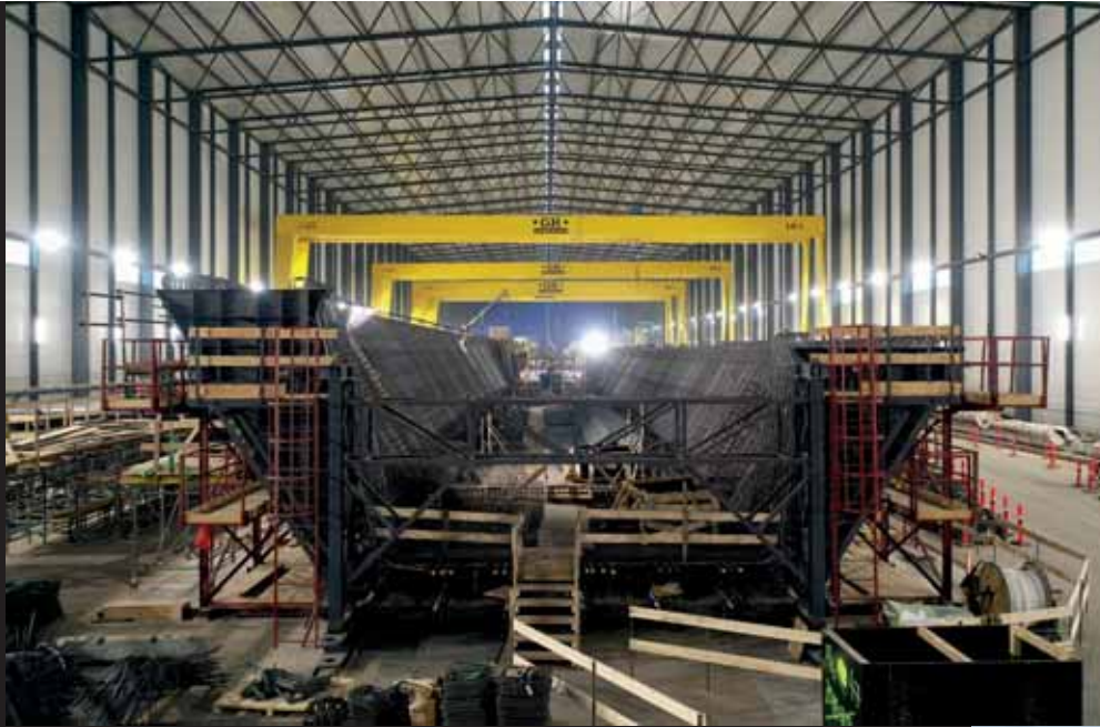
Prefab bridge deck Length approx 70 m
