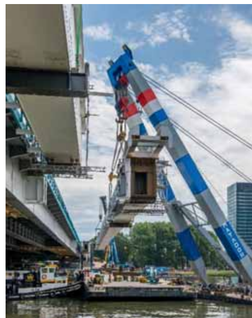
21 Inhangen VSLiggers in Galecopperbrug © Arup
