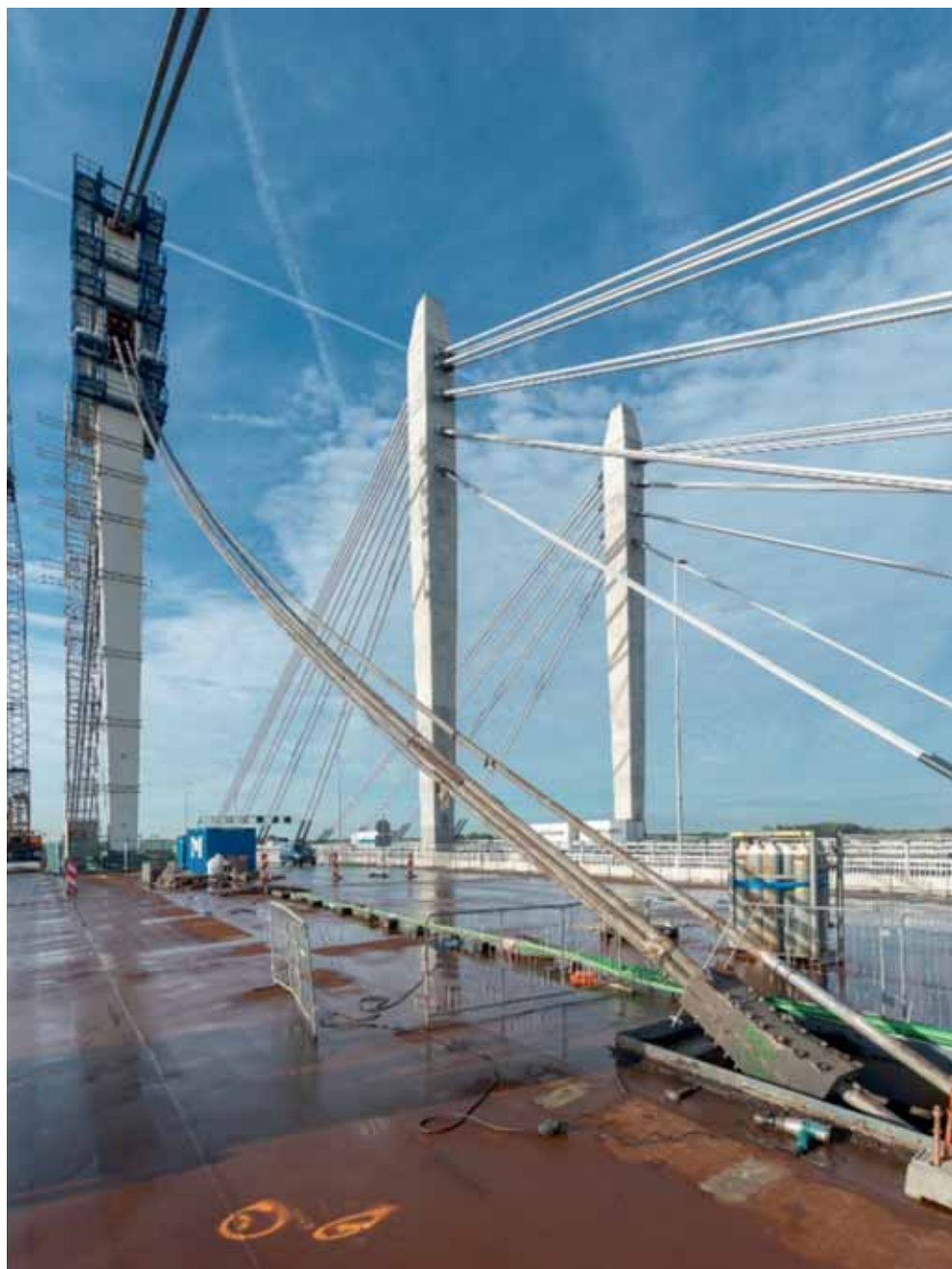
21 Inhangen VSLiggers in Galecopperbrug © Arup
