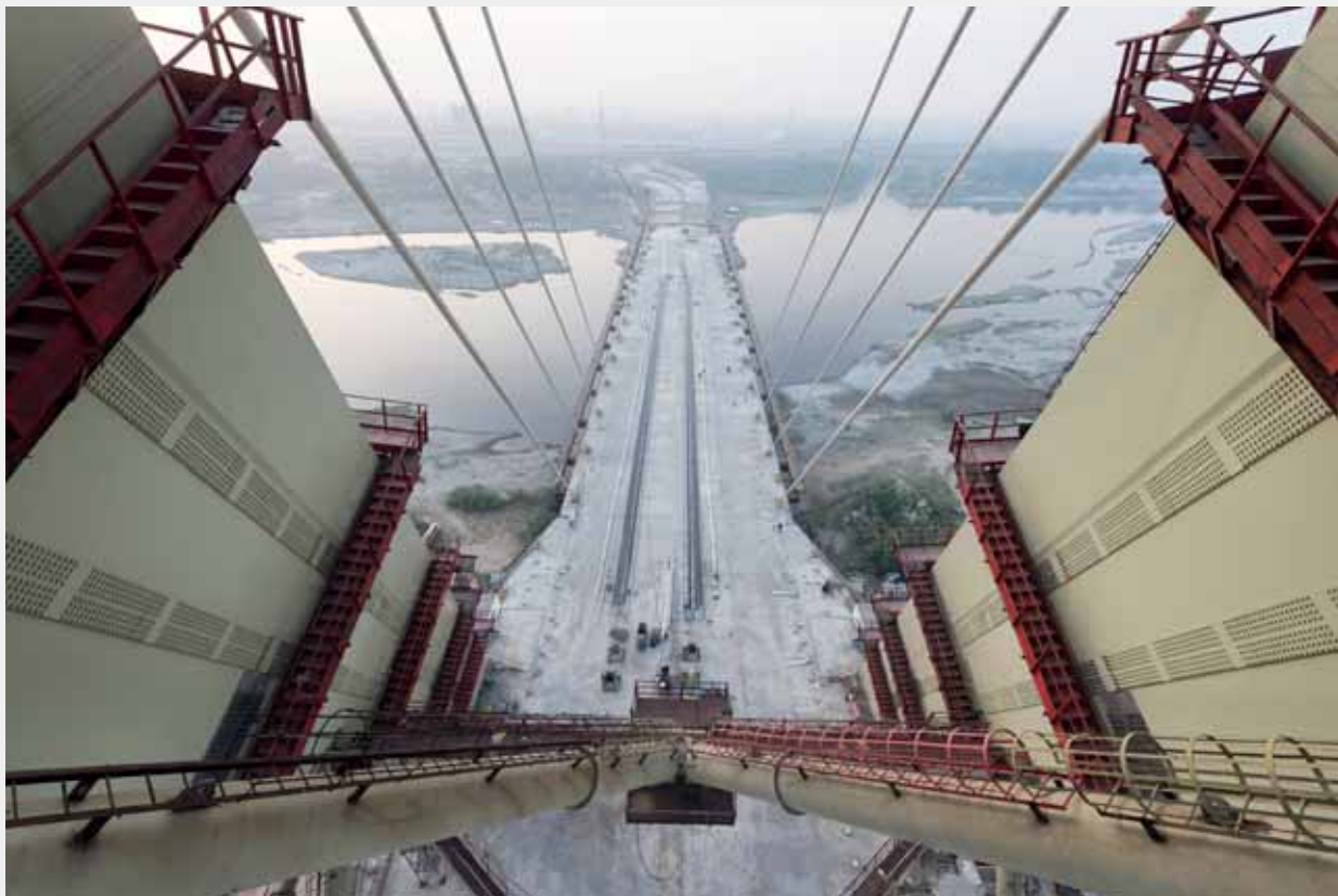
Yamuna Bridge in New Delhi nearing completion. © Andreas Deffner
